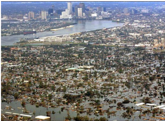
New Orleans, August 2005 after Hurricane Katrina.
